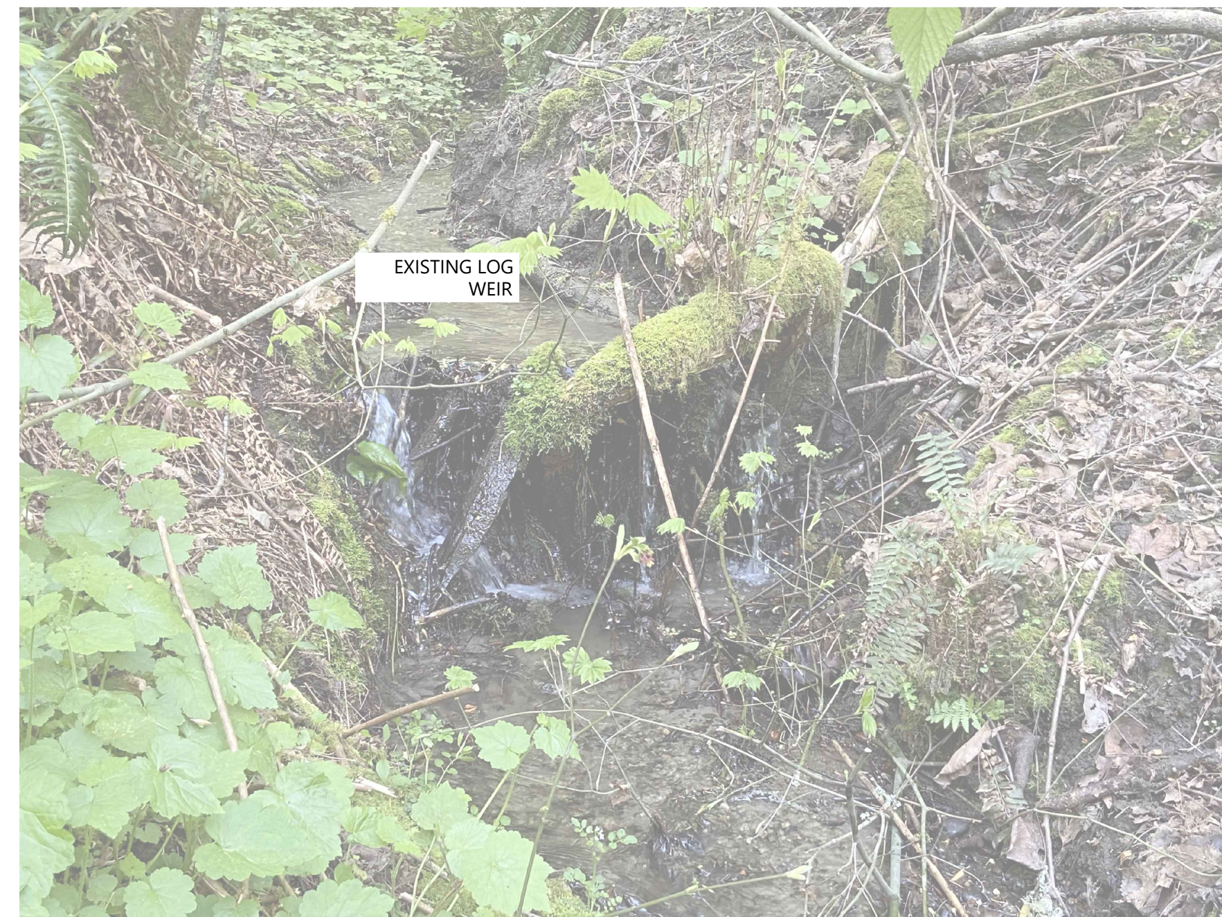
EXAMPLE PHOTO (STA 5+45)
